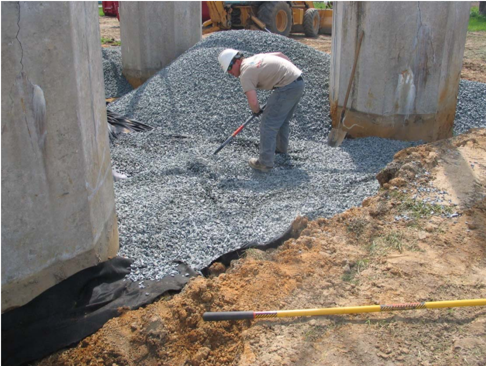
Placement and spreading of #57 type stone above filter fabric.
