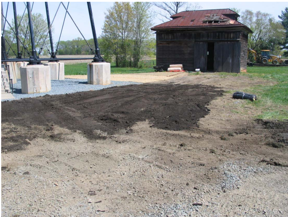
Placing additional topsoil over graded subbase to support vegetation.
