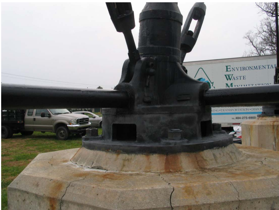
Typical condition after lead based paint removal and application of primer.
