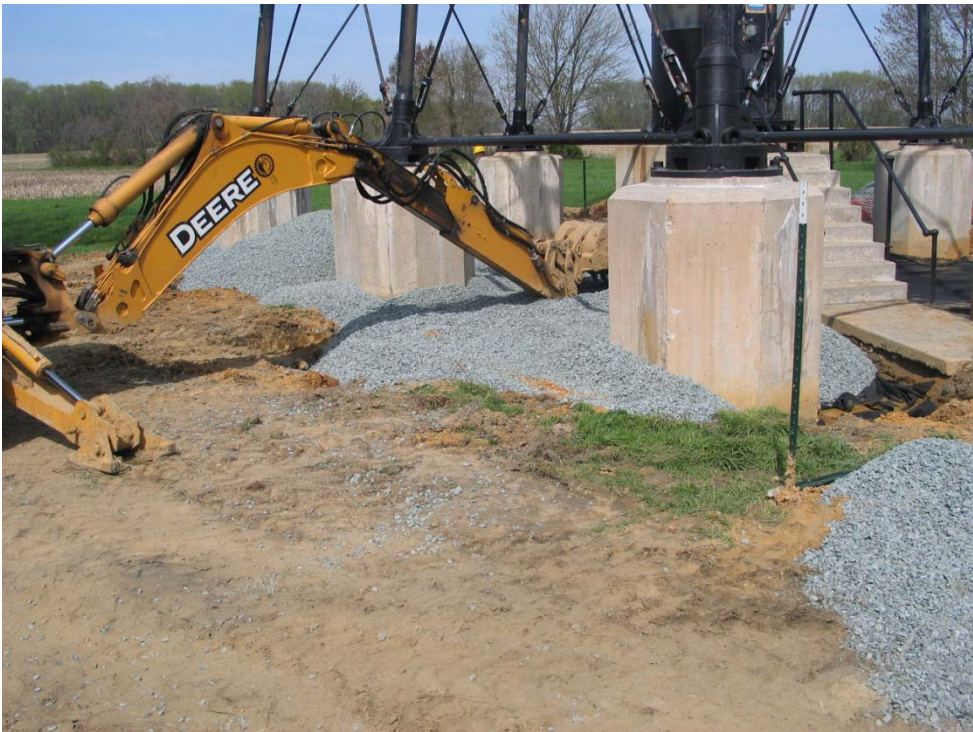
Placing backfill stone and spreading/compacting with excavator bucket.
