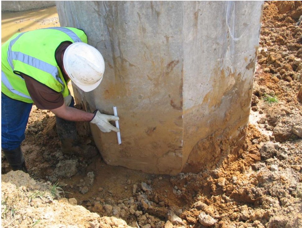
Verifying that the excavation is 2 ft below ground surface as required.
