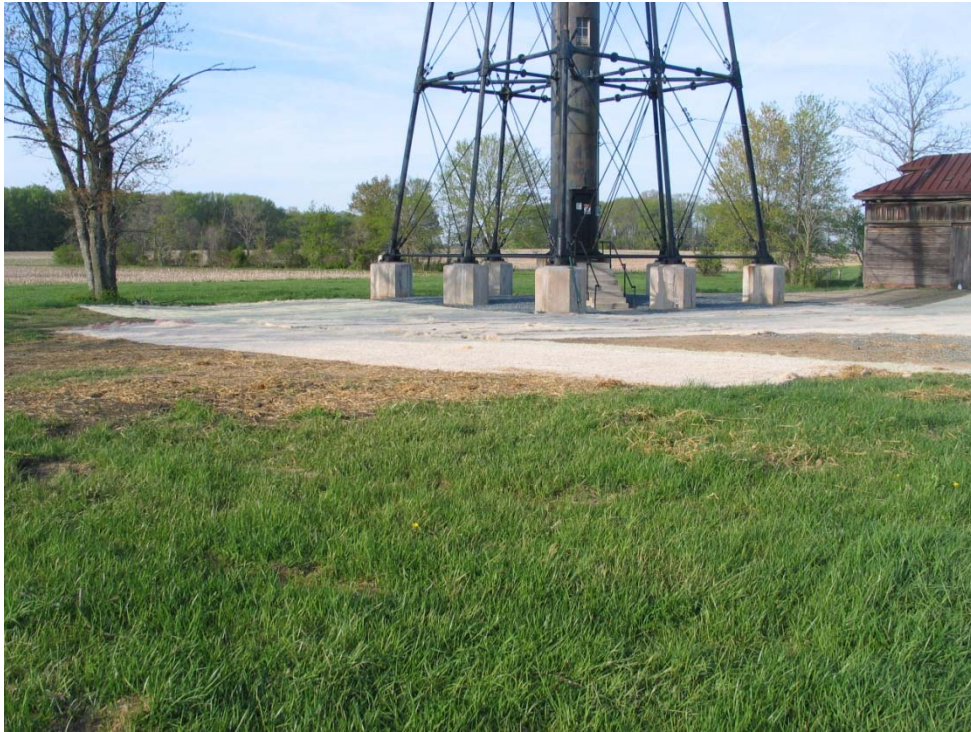
Placement of erosion matting on top of topsoil.
