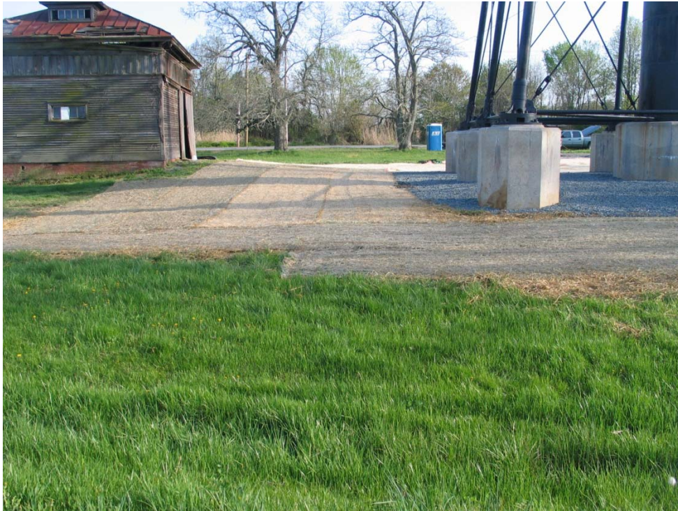
Placement of erosion matting over topsoil .
