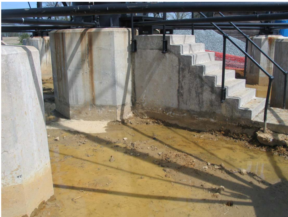
Typical conditions after excavation (2 ft below ground surface). Groundwater infiltrating excavation.
